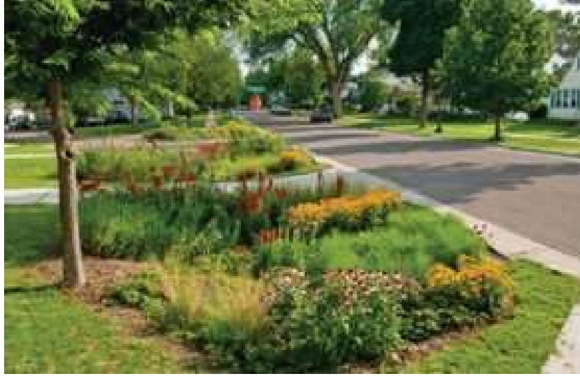
Figure 3-1: Bioretention cell in Lincoln, NE
