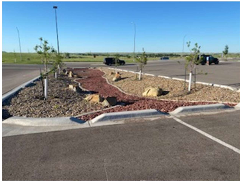
Figure 3-1: Bioretention cell in Lincoln, NE
