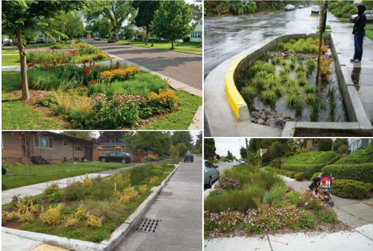
Figure 8-8: (A) Rain garden in St. Paul, Minnesota (B) Curb Extension in Portland, Oregon (City of Portland, 2012) (C). Bioretention in 34th & Cloverdale in Seattle, WA. (D) Bioretention Swale in a residential street. (NACTO, 2017).
