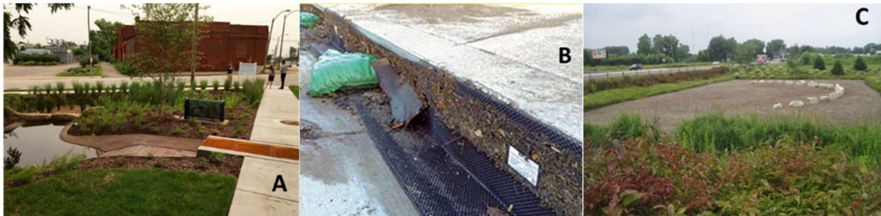
Figure 5-9: (A) Settling Device as rain garden forebay. (B) Screen. (C) Vegetated Filter Strip. (“ Overview and methods of pretreatment ,” Minnesota Stormwater Manual, 2020)
