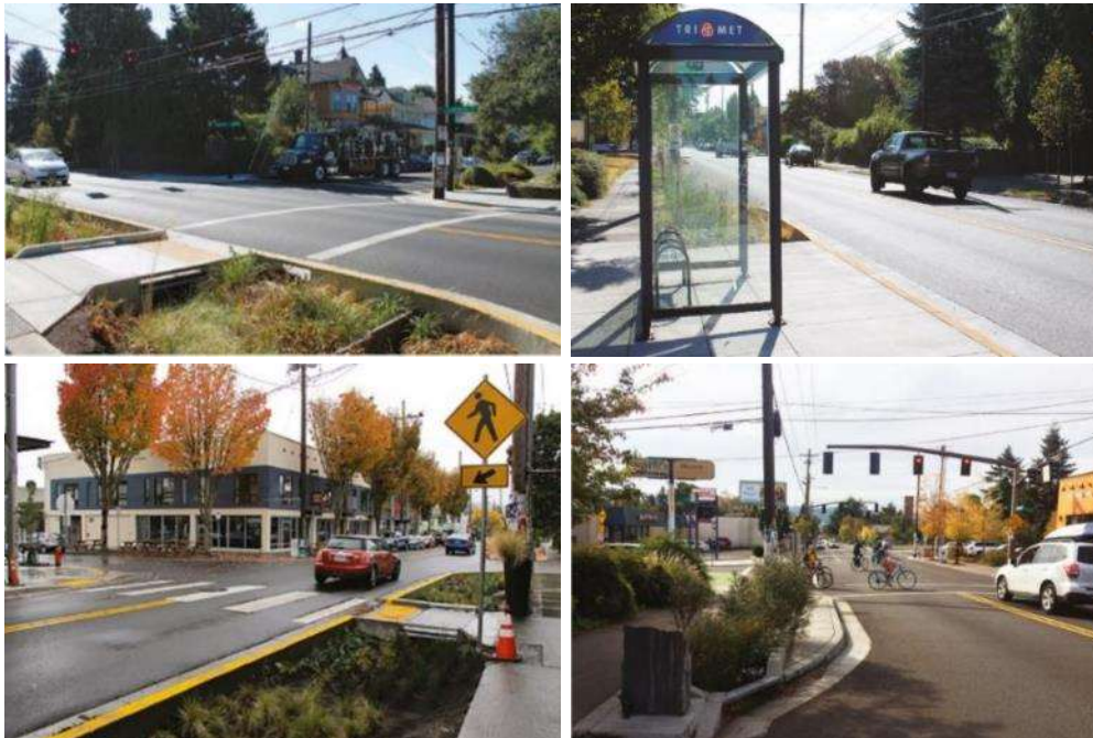
Figure 8-6: (A) T-intersection curb extension in Portland, Oregon. (B) Transit Stop in Portland, Oregon. (C) Midblock crossing in Portland, Oregon. (D) SE Division Street, Portland, Oregon (NACTO, 2017)
