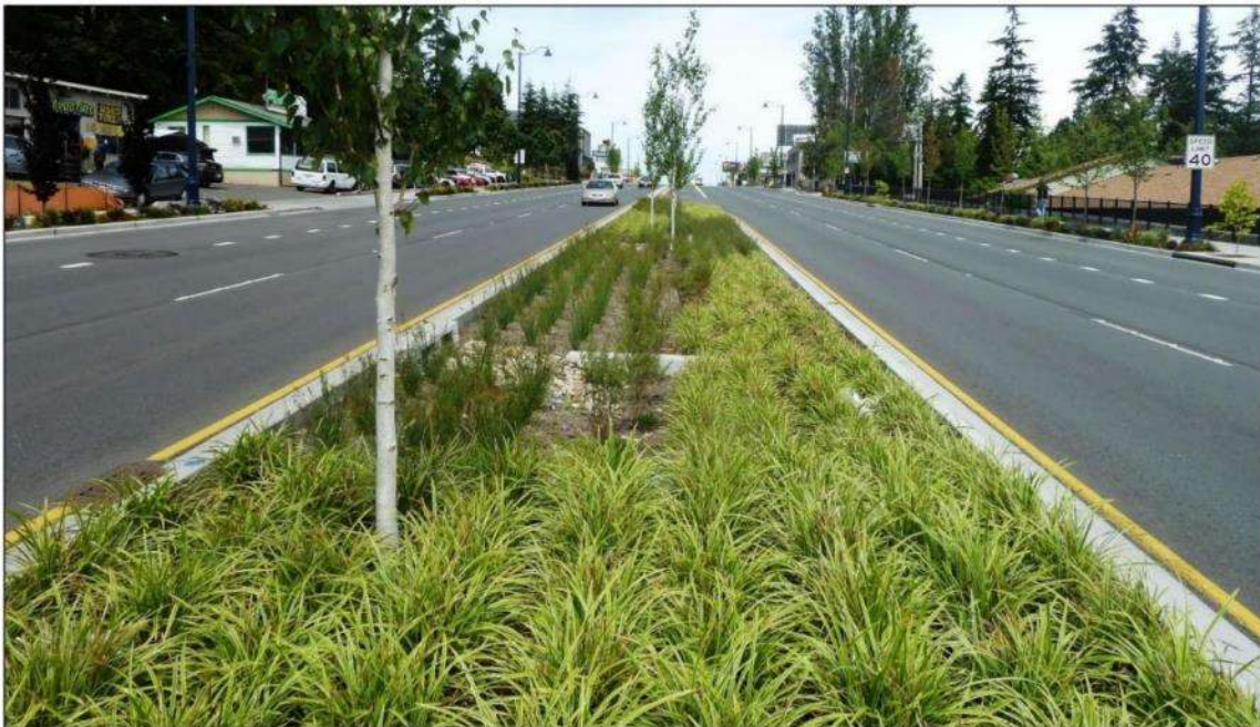
Figure 8-4: Bioretention area within roadway median (Montana Department of Environmental Quality, 2017)
