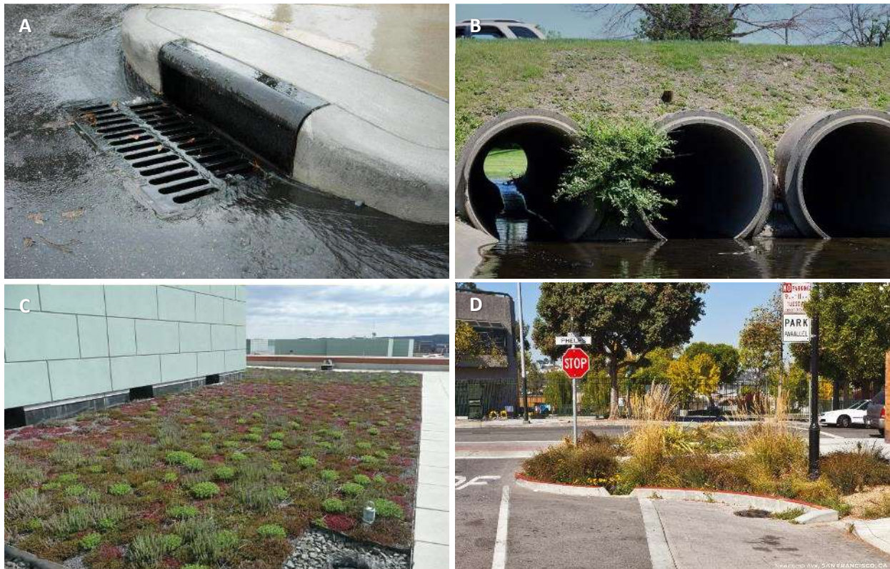
Figure 2-4: (A) Storm drain (City of Portland, 2012), (B) Culvert (“Grading a Culvert”), (C) Green roof (City of Portland, 2012), (D) Curb extension bioretention cell (NACTO, 2017).
